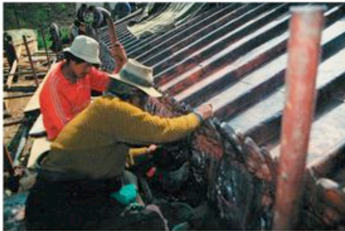
Artisans installing fascia in Tibet
